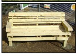
Step 5 – Install the (2) 4x4x19 ½" front legs underneath the armrests by using (2) 60D nails through the armrests. Leave 16" between the front and back
