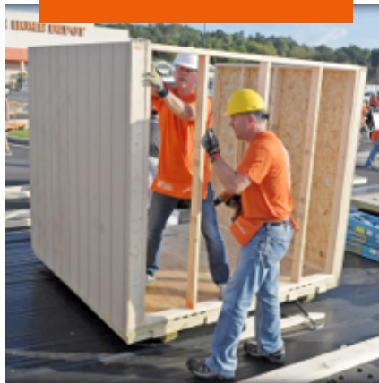
Parking Lot Builds
